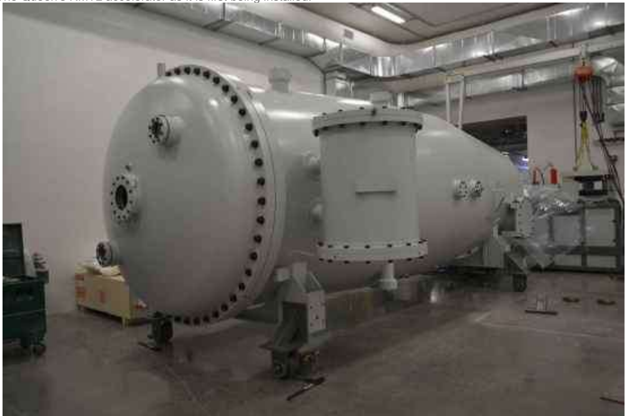
The Queen's RMTL accelerator as it is first being installed:
