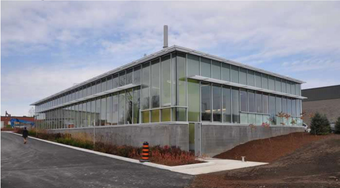
The new building
